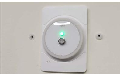
7. Careful not to kink the tubing or wire push the pressure pickup lense into the center of the front cover. It will snap it. Pay attention to orientation ensuring the Setra logo is properly oriented
