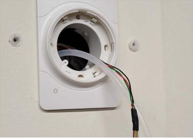
4. Thread the tubing and wire lead through the front cover and snap the front cover into place.
