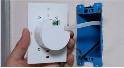
1. Connect pressure tubing from the Pressure Pickup Port to the port on the back of Setra Lite.
