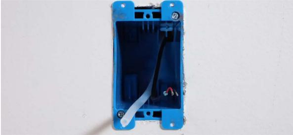
1. Cut a 2" hole in the wall for the Setra Lite base unit or install 1-gang electrical box
