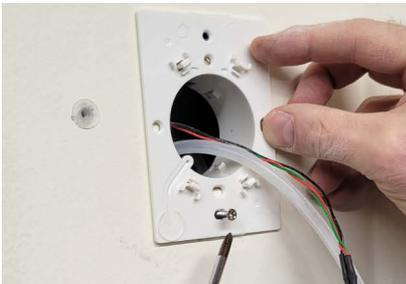
2. Secure the mounting plate with provided mounting hardware based on installation type (Direct wall or electrical box)
