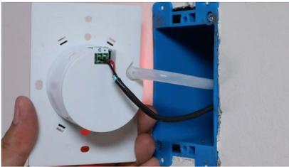
2. Connect wiring for power and analog output (if required) per section 7.0 Dual Alert: This variant will have an additional wire lead connected to the back of the unit. Thread the wire lead through the wall and into the pressure pickup port box or hole on the opposite side of the wall.
