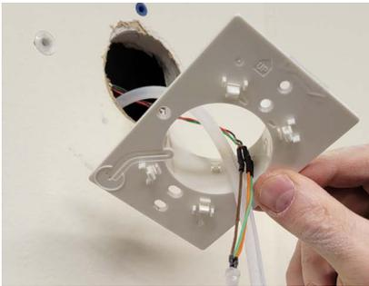
1. Thread the tubing and wire lead through the mounting plate.
