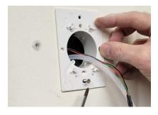
2. Secure the mounting plate with provided mounting hardware based on installation type (Direct wall or electrical box)
