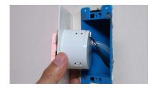
3. As you push the Setra Lite unit into the electrical box, push the tubing into the conduit tube or into the wall cavity.
