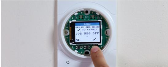
Press and hold the RIGHT button ("✓") to adjust the room pressurization (i.e. whether the room is positively or negatively pressured); the screen text will flash 3 times to indicate that the setting is ready to be adjusted.
