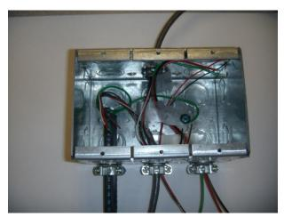
Fig. 3-4 Rough Plumbing and Wiring to Rough-in box, Flush Mount Unit
